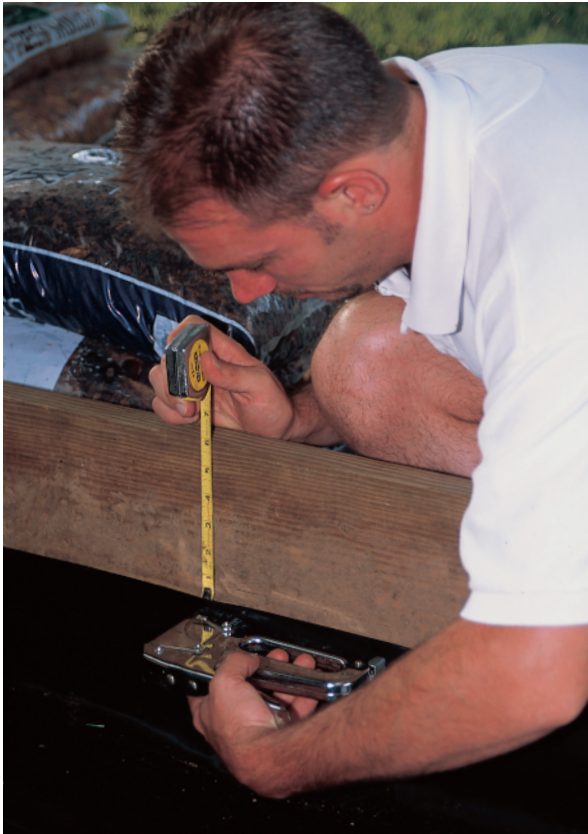
Line the frame with plastic, stapling it in place.
