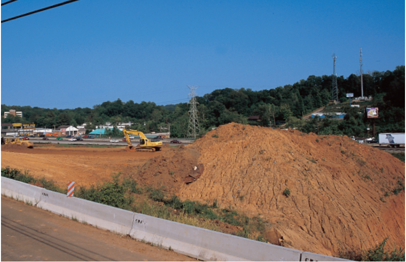
Construction along Interstate 40 near Knoxville, Tennessee, typifies the most significant threat to native plants: habitat destruction.
