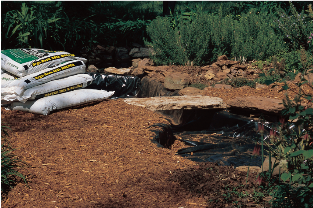
Constructing an in-ground bog bed requires digging, and lining the excavation with heavy plastic.
