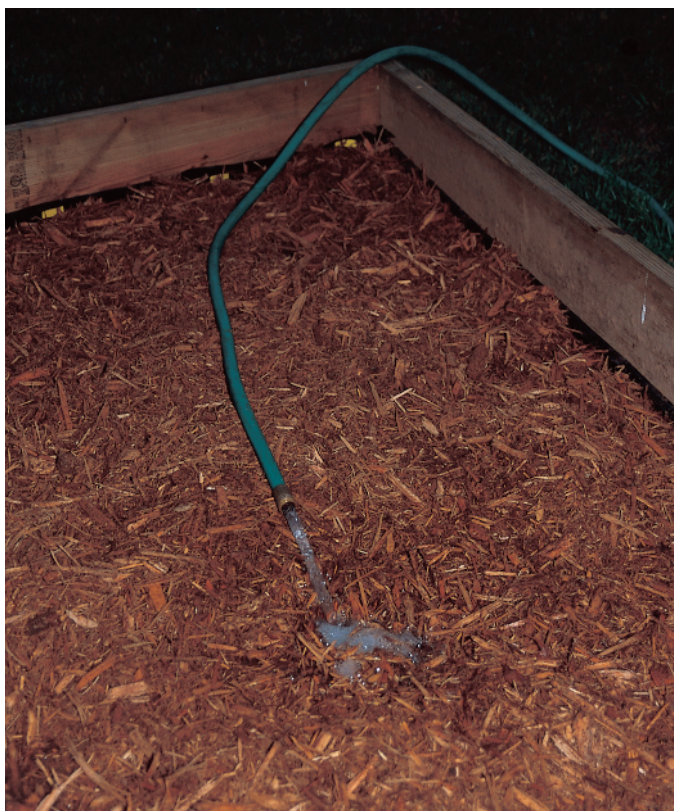
Flood the filler material with water and allow it to soak overnight before proceeding with construction.
